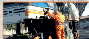
Road milling/fresature stradali
